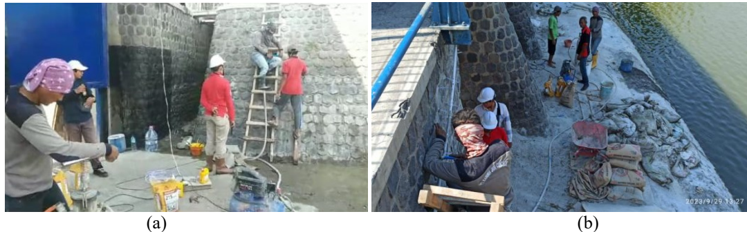
Figure 13. (a) grouting process of the stone masonry wall and (b) grouting process of the floor
