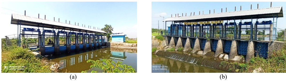
Figure 1. (a) Front view and (b) back view of the Tinggar Buntut Barrage Mojokerto
